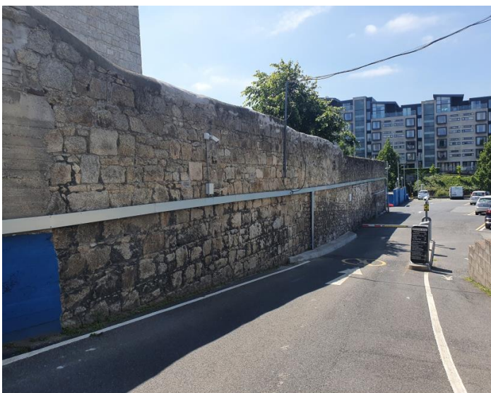
3. Northern Boundary Wall with Parochial House
