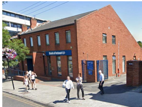
2/3 Main Street (Bank of Ireland)
