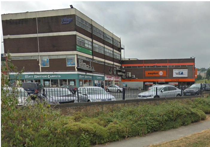
14. View of Rear of Dundrum Village Centre from Bypass
