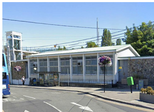
EIR Telecom Exchange, Main Street
